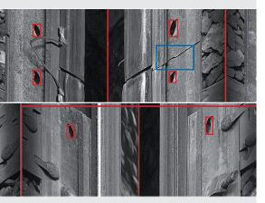
Broken fishplate / joint bar; missing bolts
